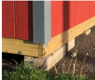
Figure 2 - Close-up of leveling with blocks & shims
