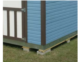
Figure 3 - Display building with wood skids beneath the floor joists
