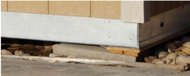
Figure 2 - Close-up of leveling with blocks & shims
